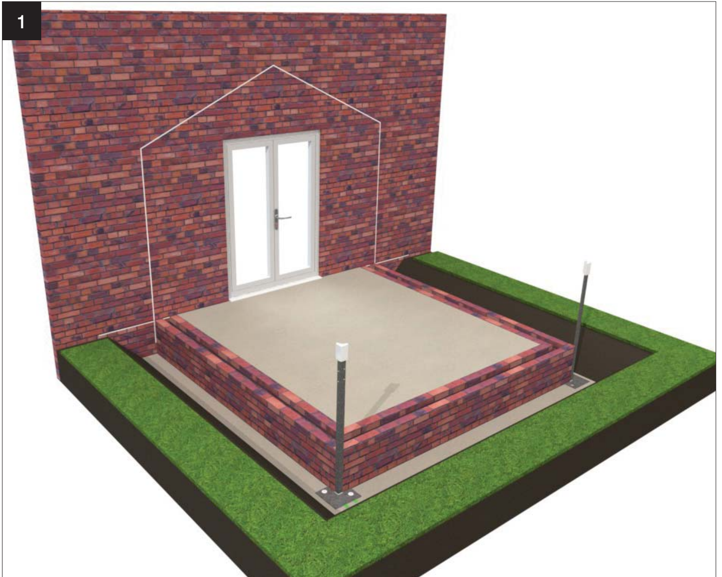
Foundation set out posts (There are 2 types of set out posts that may be ordered / specified)
