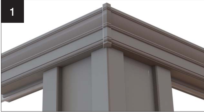
Loggia with Cornice
